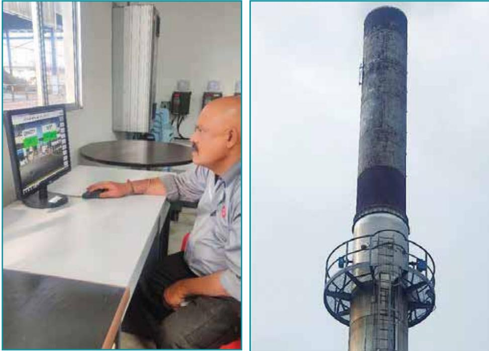
Figure: Biomass Boiler Monitoring system. Left: Personnel monitoring the biomass boiler system in the boiler room, Right: CEMS system to be installed at the biomass boiler chimney stack to monitor dust particulate emission.
